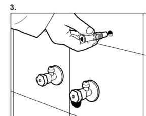
3. The marked places are drilled. Stop are placed.
